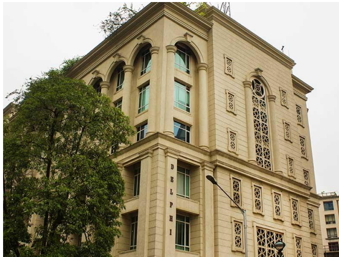
Building where TANAKA KIKINZOKU (INDIA) Private Limited is located
