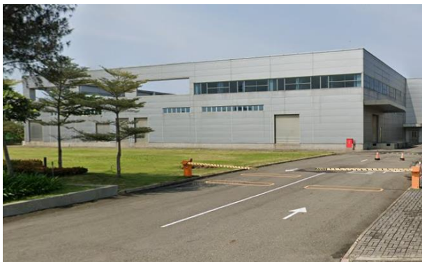
Exterior of new plant
